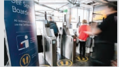
Biometric airline gate turnstiles will allow passengers to directly board a plane without showing a ticket
